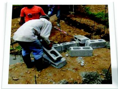
Left: Young people laying the first line of block on the freshly poured foundation. Middle: Elizabeth tries to work with the wheel barrel for a moment. Right: The breathtaking view of the cloud filled valley below Beautiful River at 6:15 am.
